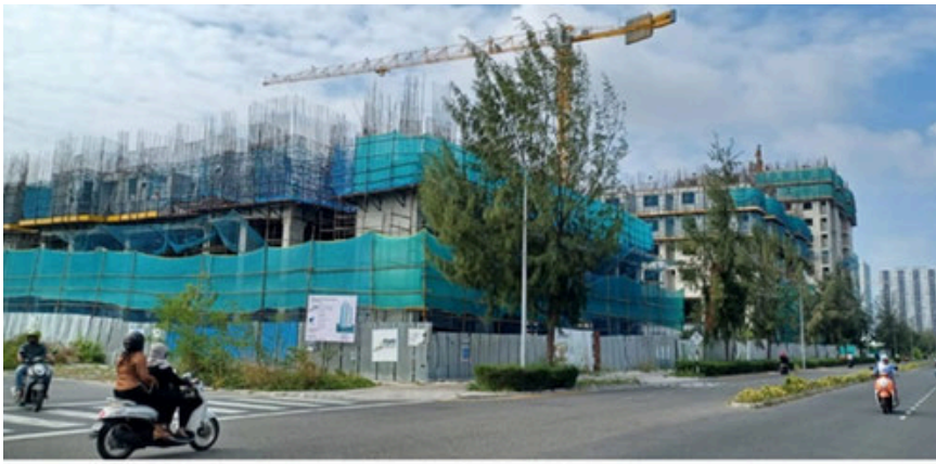
Dust screen arrangements were implemented at the ongoing construction site in 2023.
